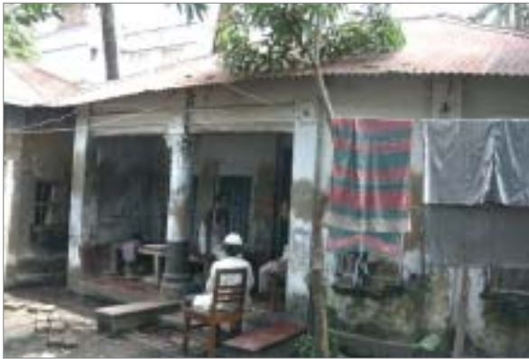
Figure 5.32: View towards the main living unit from inner court. The activities at the veranda are similar to a vernacular house.
