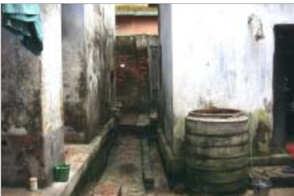
Figure 5.37: The approach towards the detached toilet.
