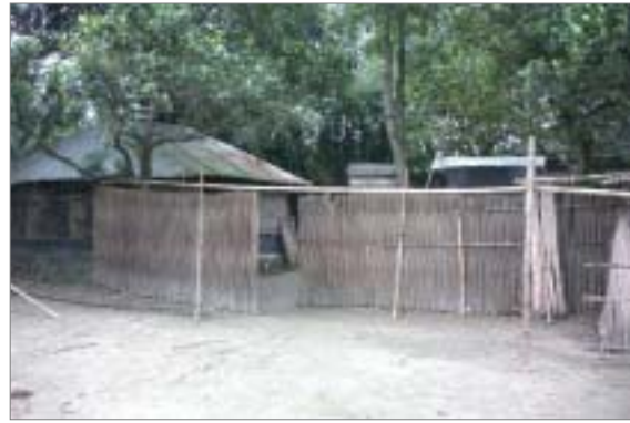
Figure 5.16: The indirect approach to the inner court. Fences are made with jute sticks.
