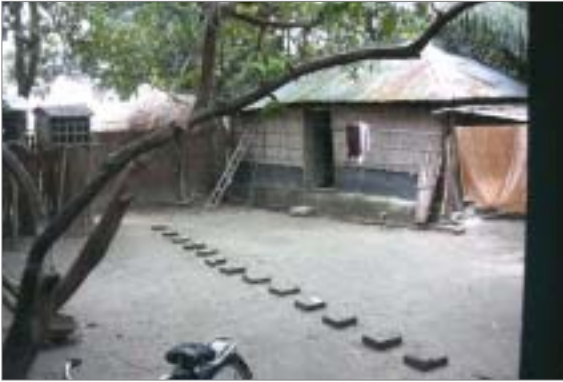
Figure 5.15: The inner court. Trees, built forms are making the environment cool and private.
