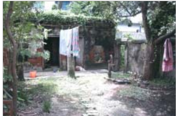
Figure 5.33: View of the inner courtyard showing the detached kitchen (now abandoned).
